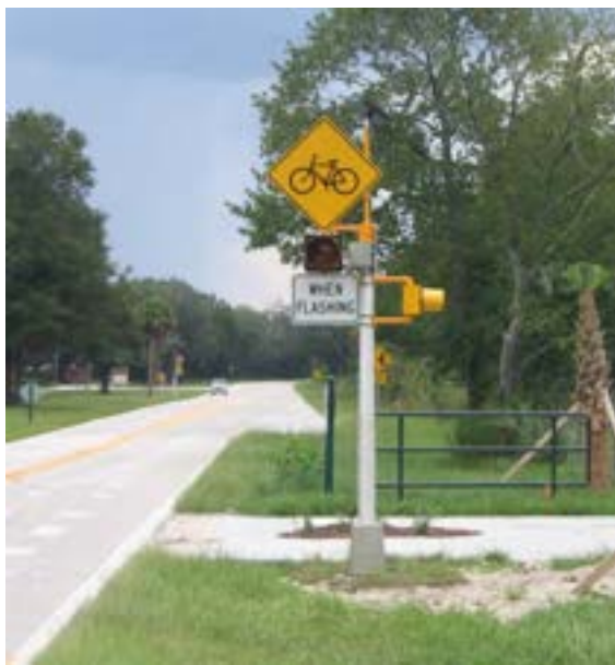
Fig. 9.7G. Active Crosswalk Warning Systems
