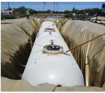
This compartment tank includes 2 bulkheads, an alternative in this limited space to installing 3 individual tanks.
